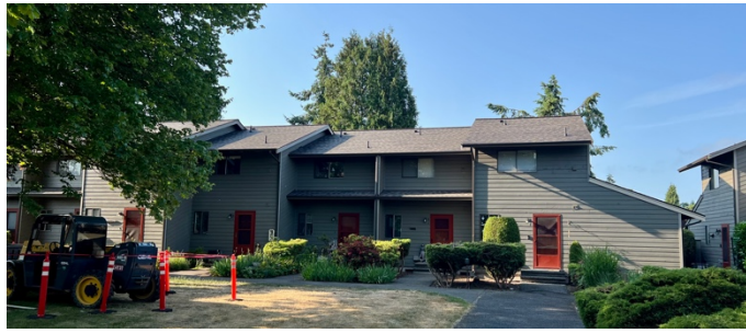
Birch Building Gets a New Roof!
